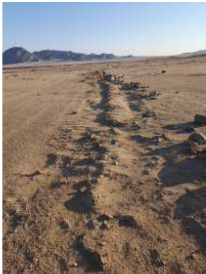
Existing pipeline looking North towards the Roessing pipeline
