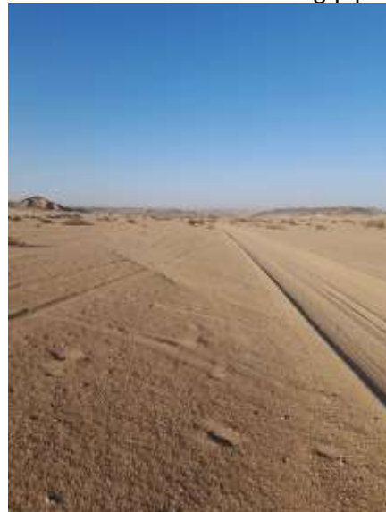
Existing pipeline looking North just before it goes into the Swakop River to Farm Weizenberg
